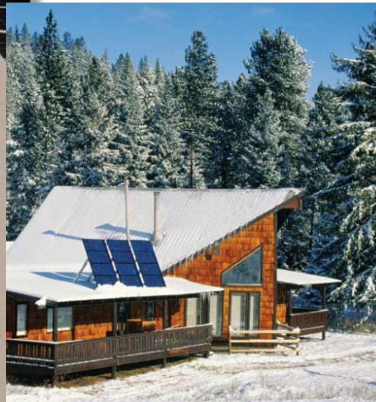
↑ This home has solar panels on the roof to provide power.
